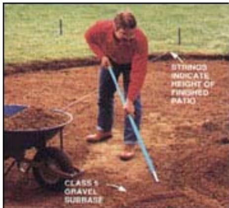
**4. SPREAD CLASS 5 subbase to a depth of 4 inches over entire patio area and 8 inches beyond. Measure down from guide strings to establish uniform height of subbase.**
