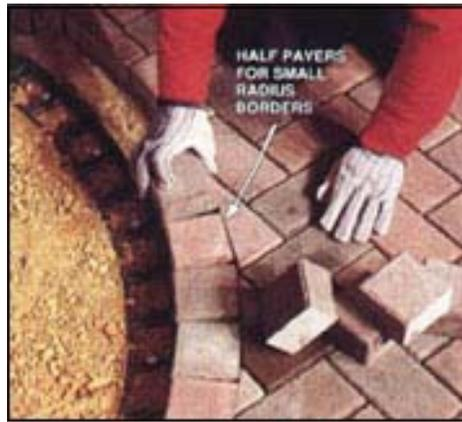
12. **USE HALF PAVER** for bordering tight circles. Smaller pavers cut down on the size of the pre-shaped gaps between each piece.
