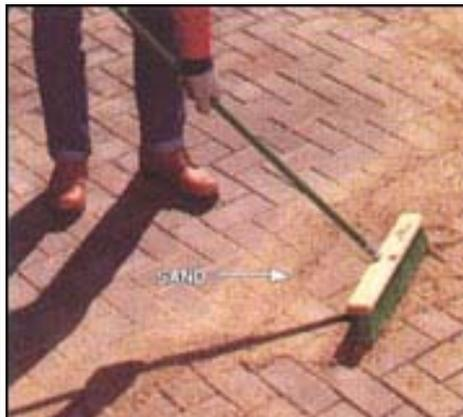
15. **SWEEP COARSE, DRY SAND** between cracks of pavers to lock together and fill voids. Repeat with more dry sand in a few days.
