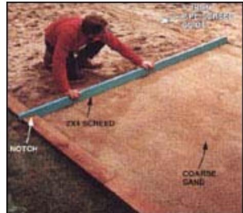
8. **SPREAD AND LEVEL** a 1 inch bed of sand over compacted subbase. Pipes provide a guide for dragging the 2x4 screed board across.
