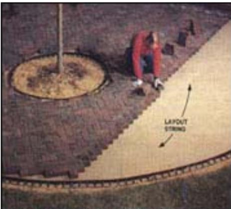
**10. CONTINUE LAYING PAVERS** using a layout string to keep them in line as you work. Put a gap between pavers or tap them tighter to stay in line.
