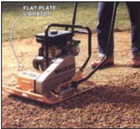
5. **TAMP THE SUBBASE** using a flat-plate vibrator (rented at \$40 a day). Work in a circular motion and compact the area twice.
